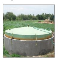
Community bio-gas plant based on cattle manure, food or agro-waste can be used for cooking or process heating. In our system, Bio-gas is distributed to the community and the usage is metered and charged to the consumers based on a predetermined tariff rate which can take care of O&M costs.
